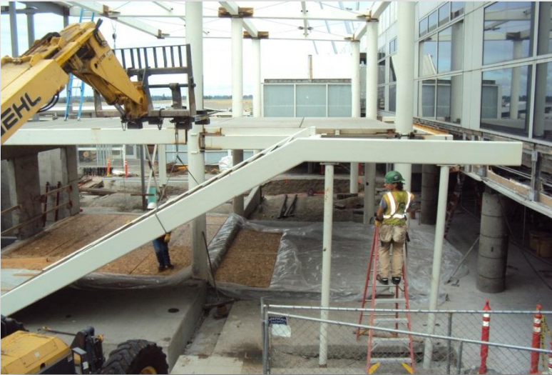
C2 Structural Steel Erection
