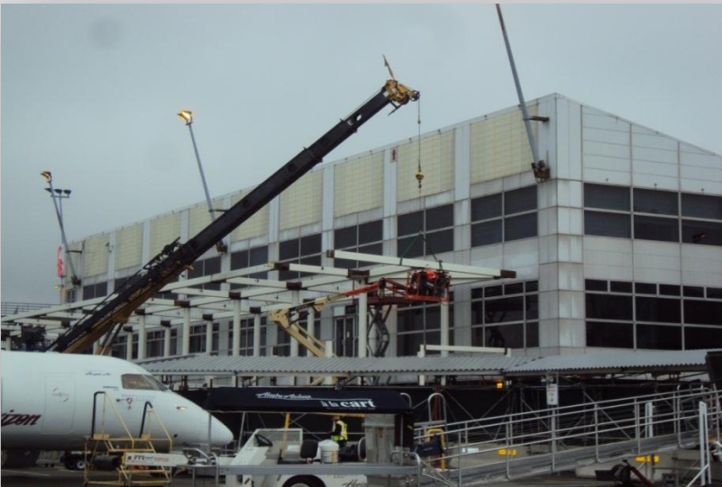
C16 Steel Erection
